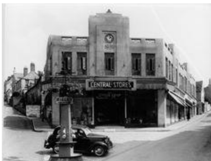
The Co-operative Building, Stroud 1930s
